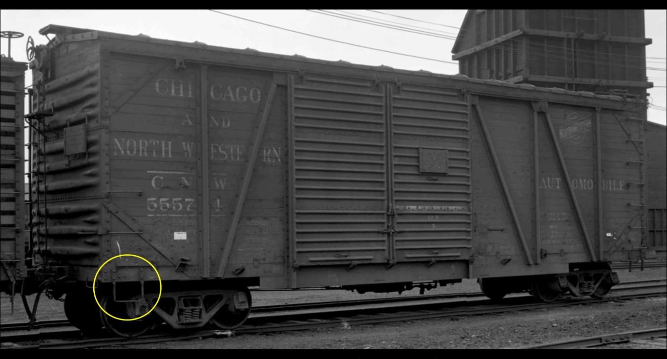
The CNW used a distinctive Sill Step that has to be fabricated if it is to be modeled.
